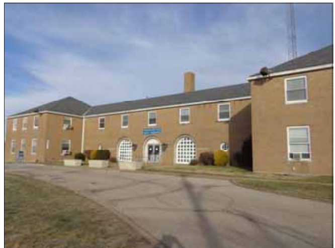
4. View of the northern side of the structure.
