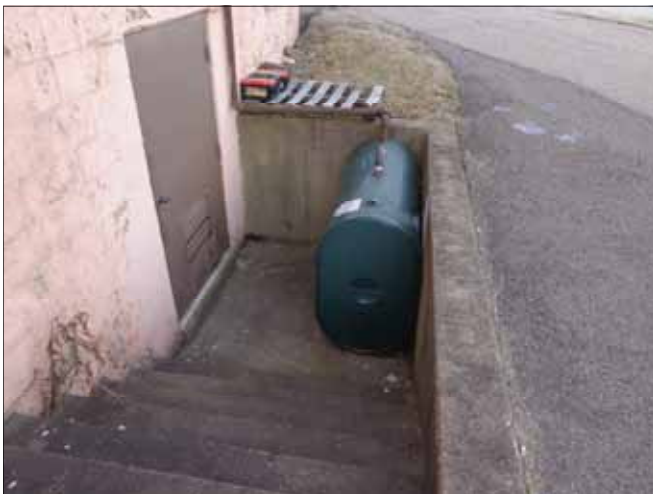
9. View of a 275 used oil AST.
