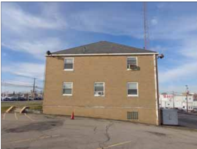
3. View of the eastern side of the structure.
