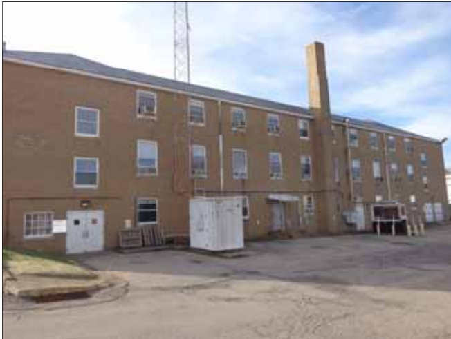
1. Looking north at the structure.
