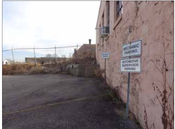
8. View of the northern side of the automotive garage.
