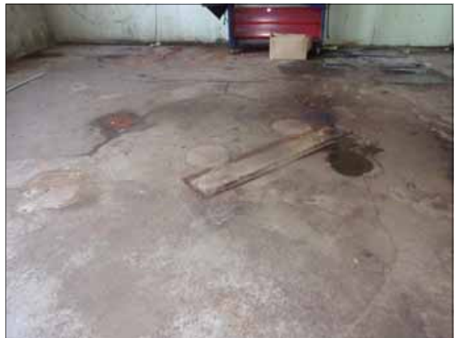
22. View of a former hydraulic lift area.
