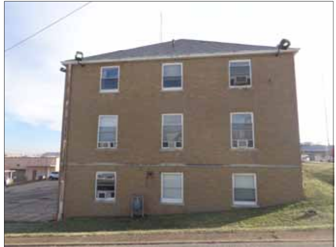
2. View of the western side of the structure.
